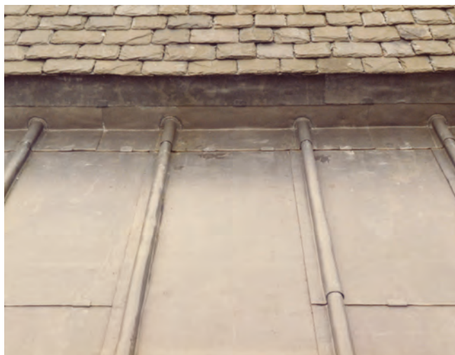
Fig 240. Abutment finishes (30° and above)
