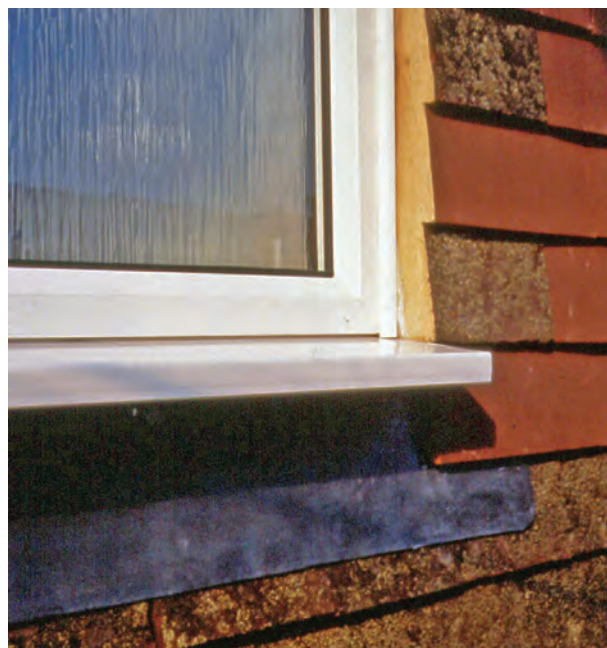
Fig 134. Sill and jamb flashings in slate hanging
